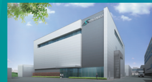
Conceptual image of new research and development building (tentative name) at Yokohama Operations
