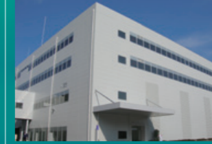
Plant building at YOKOHAMA Operations
